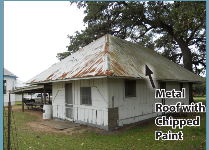
FIG. 46: Metal roofs last a long time if they are painted regularly.
