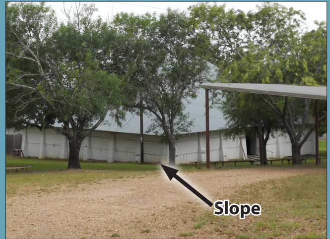
FIG. 56: Downhill slope to corner of dance hall will cause problem of pooling water against building.
