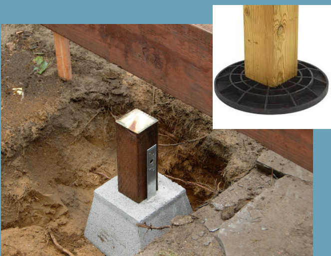
FIG. 26: Examples of replacement posts
