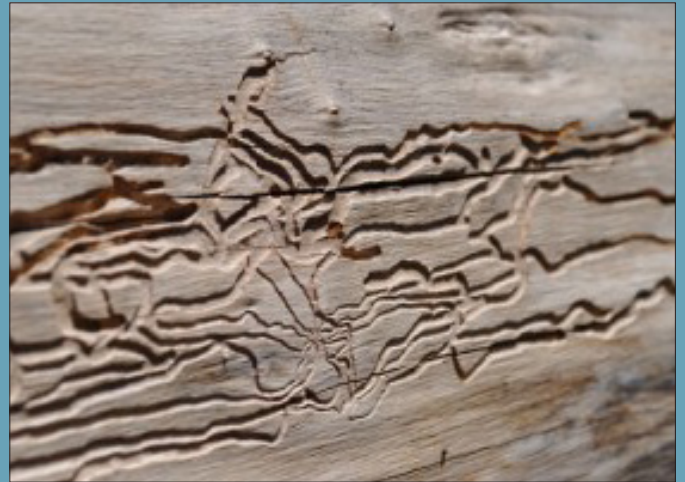
FIG. 6: Termite paths in wall.
