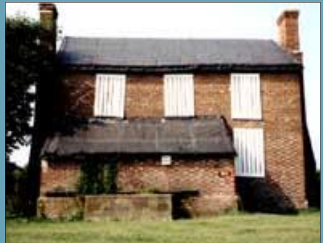
FIG. 63: Mothball - exterior. Note semi-permanent covers over window openings and caps on chimneys.
